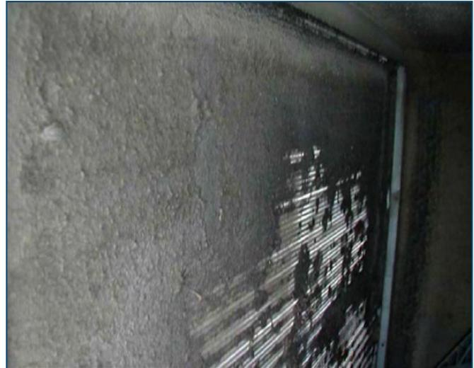
**Filthy Cooling Coils Restricting Airflow and Cooling Effectiveness. Closer inspection revealed missing air filters.**
